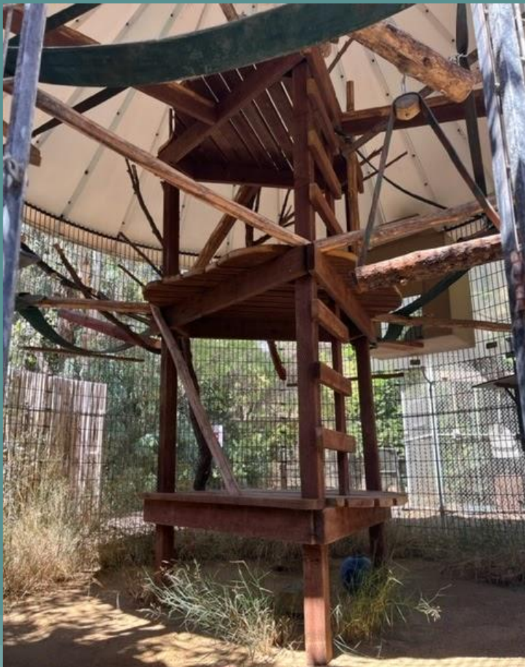
Tower, Pressure Treated Lumber
